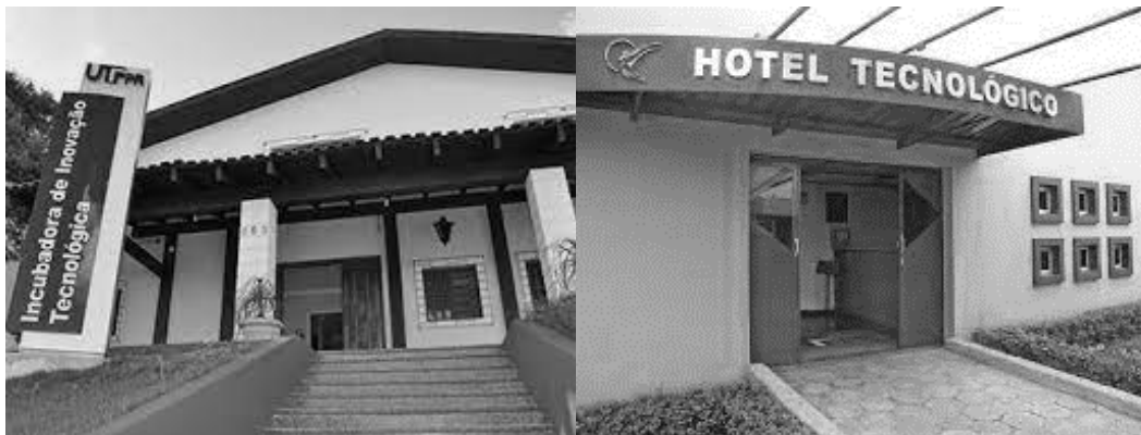
Figure 3 Frontages of the TII and TH
