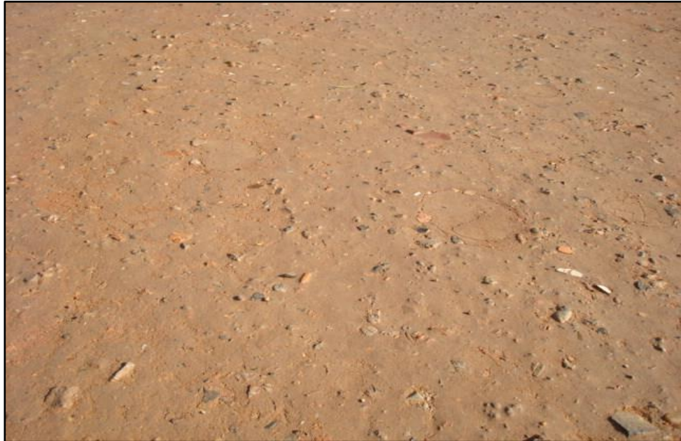
Figure 6 - Compacted material used in the recovery of public roads
